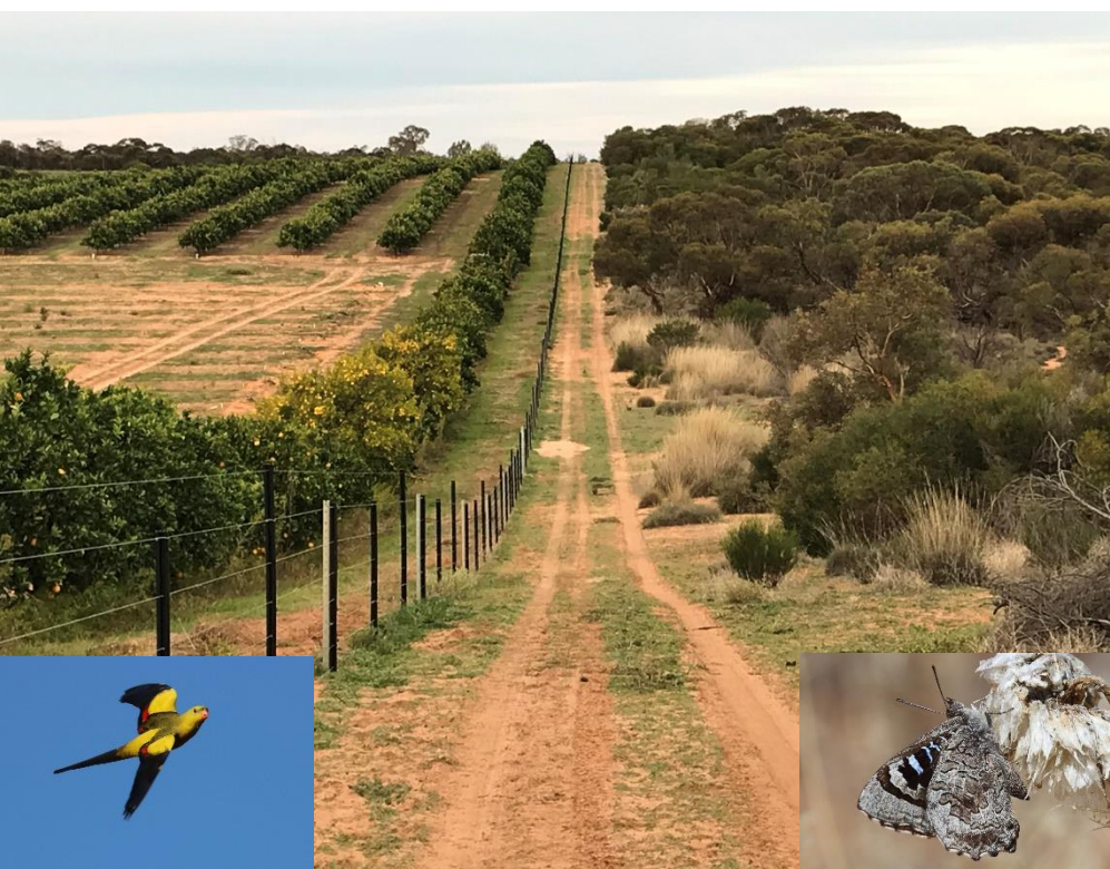
Photo (left): Raakajlim fenceline 2020. The Westonfence uses standard steel posts at 10-metre spacings with plastic (HDPE) suspension droppers between and clipped to each steel post. The plastic droppers act as insulators. Inset - The threatened Regent Parrot (left); The threatened Arid Bronze Azure butterfly is at risk from soil disturbance from pigs; (right) The Murdoch family preparing the fenceline for the new Westonfence.
