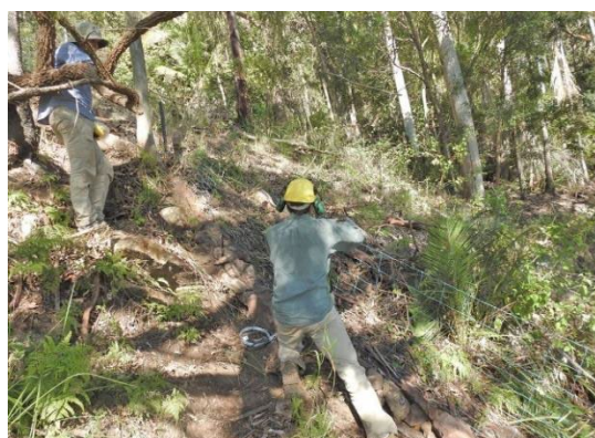
QFS volunteers constructing the pig exclusion fence Credit: QLD Frog Society
